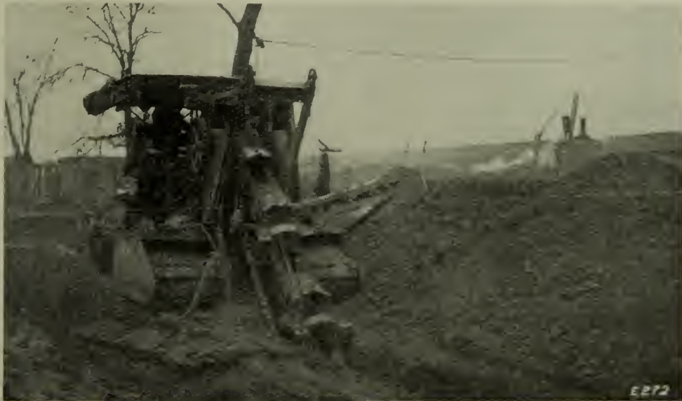
FIG. 8. A PETROL-DRIVEN MACHINE EXCAVATING TRENCH FOR A WATER MAIN.
